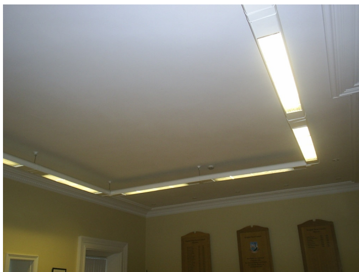
Figure 3.6 Old T12 fluorescent lighting in the council chambers
