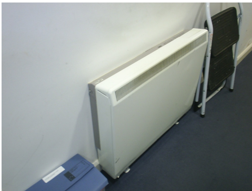
Figure 3.3 Storage heater in office area
