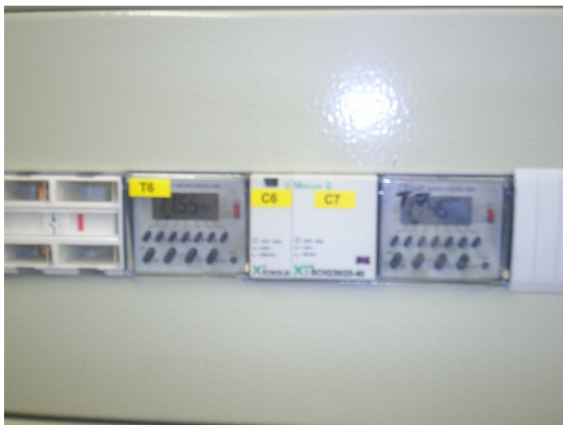
Figure 3.5 Timers on immersion heaters
