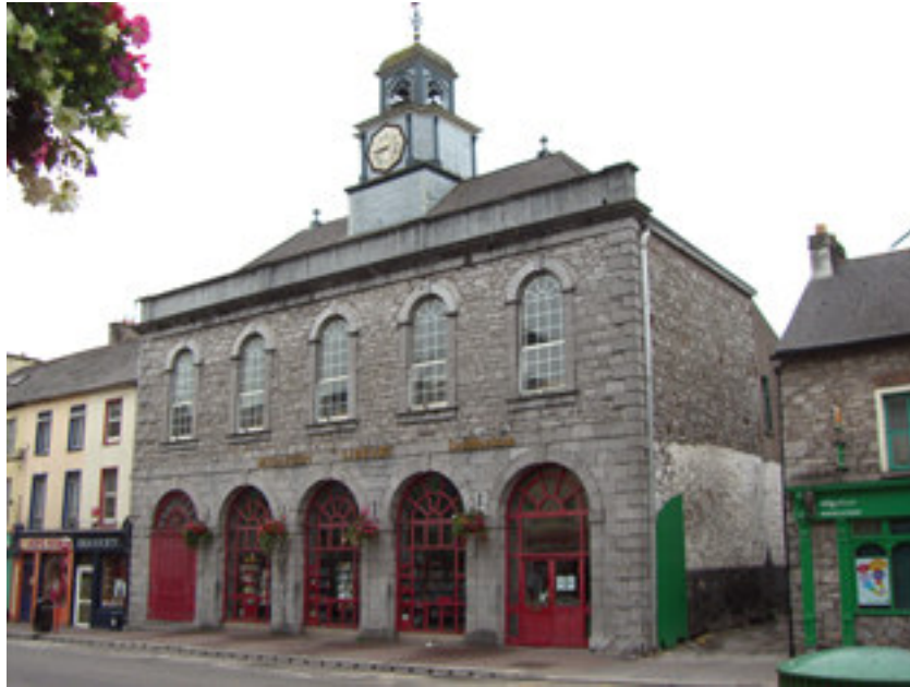
Figure 2.1 Midleton library building
