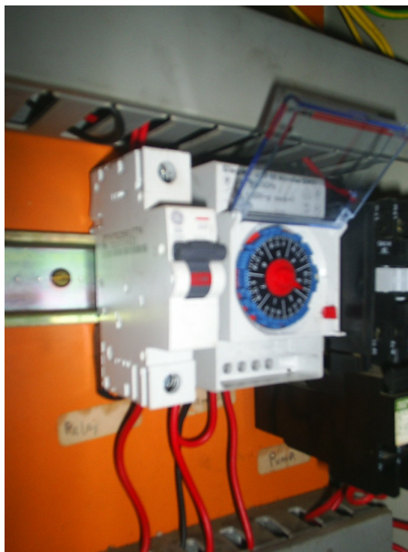
Figure 3.5 Seven day timer to control boiler
