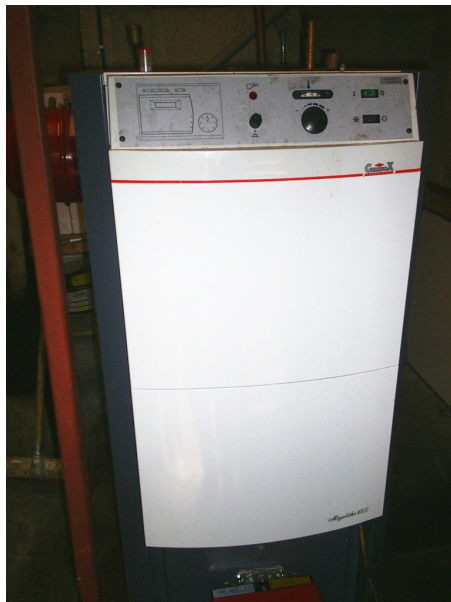
Figure 3.3 Main oil boiler
