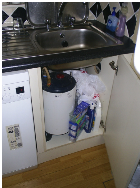
Figure 3.6 Electric under sink heater in kitchen
